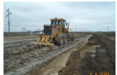
Lime Stabilization Process
